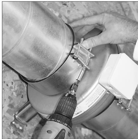
**3.** Strap the duct clamps on each side of the fan with the screws.
