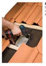
**ENG:** Mount the underlay seal onto the wood through the underlay with screws. If the underlay is made of plastic and there is no wood under it, put the underlay seal under the plastic, so that the spikes go through the plastic. Press the plastic tightly against the silicone and screw down the screws in the upper and lower battens.
