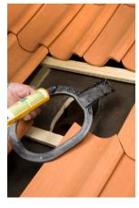
**ENG:** Put rubberized bitumen sealant on the bottom surface of the underlay seal, if the underlay seal is made of bitumen. If the underlay is made of plastic, put silicone sealant on the top surface of the underlay seal at the place where there are spiked pins.
