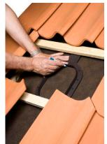
**ENG:** Mark a hole in the underlay by using the underlay seal. The seal must be attached to the lower batten.
