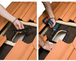
**ENG**: Attach the bracket to the side of the lowermost batten with two long screws. Check that the sideways location is correct.
