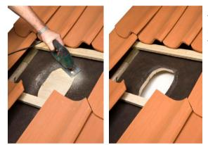
**ENG:** Make a hole of the size of the drawing in the underlay. If there is boarding under the underlay, cut a hole in it that is the same size as the hole in the underlay.
