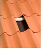
**ENG:** Remove one tile to which you will install a Universal tile pass-through. Make sure there is not a roof truss at that spot.
