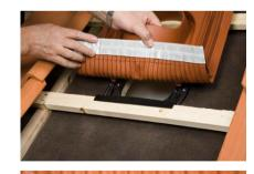
**ENG:** Now you can remove the tiles located next to the hole, so that you can install the pass-through on the long pins of the bracket. If the batten spacing is too close, you may have to make cuts in the batten on the topside, so that the cowl of the pass-through can fit between the battens.
