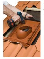
**ENG:** Mount the top part of the pass-through onto the batten with two short screws. Choose an appropriate seal of the three seal alternatives for the top edge of the passthrough. Remove the protective film of the tape from the pass-through, and mount the seal onto it. Make sure that it is in the correct location sideways.
